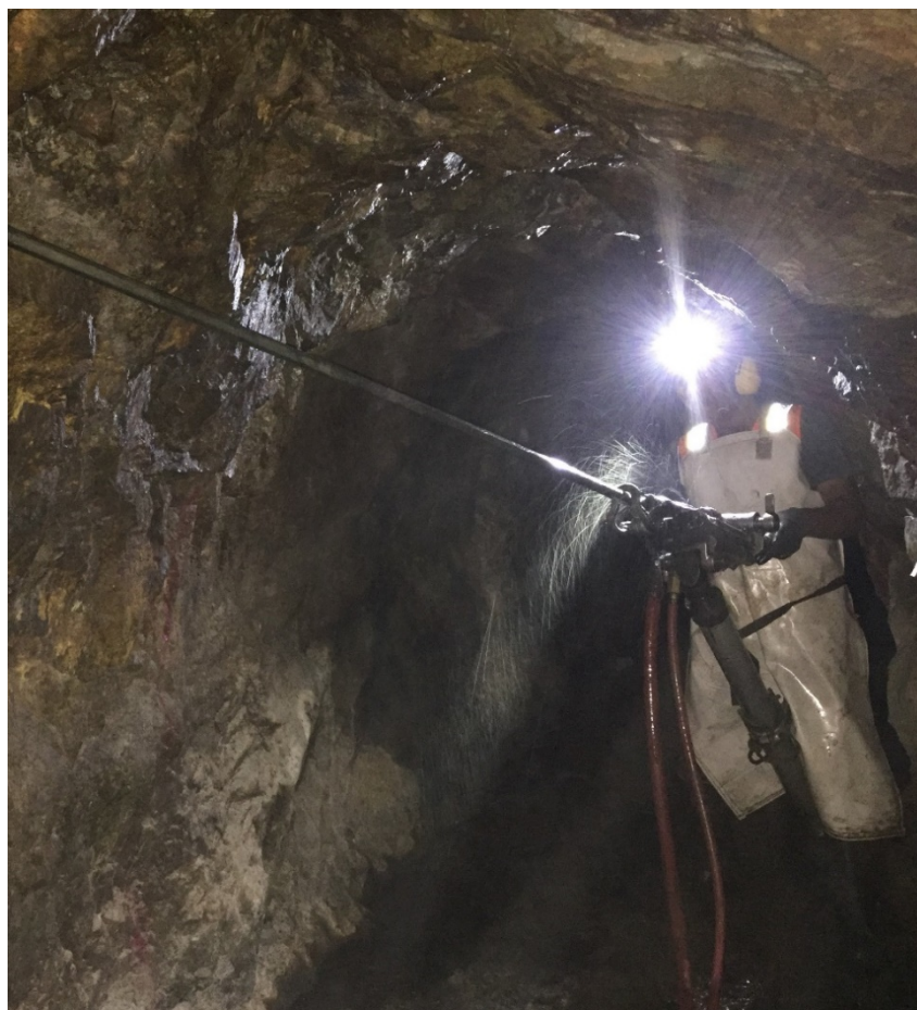
Figure 4: Drilling blast holes to expand underground tunnel (T-001) at San Marcial
