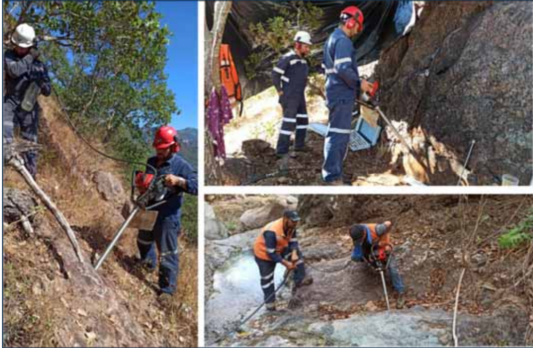
Figure 10-28: Adapted Portable Drill Rig to Difficult Access Areas at Surface
