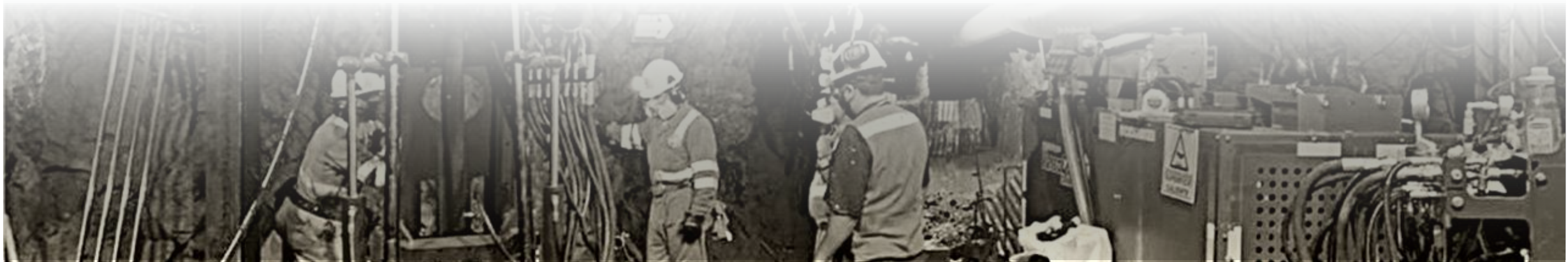
Underground Drilling San Marcial Tunnel
