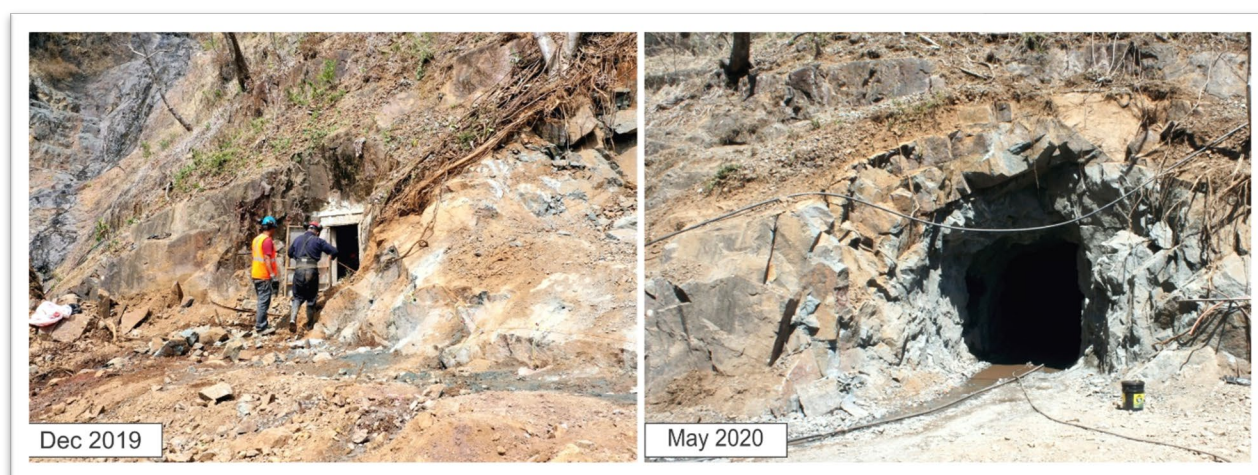
Figure 5: San Marcial Tunnel - Underground Development in 2020
